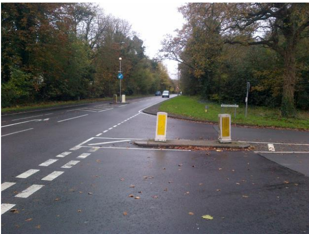
Image 5 – View to the right from Rangers Road (taken on 13/11/14)
