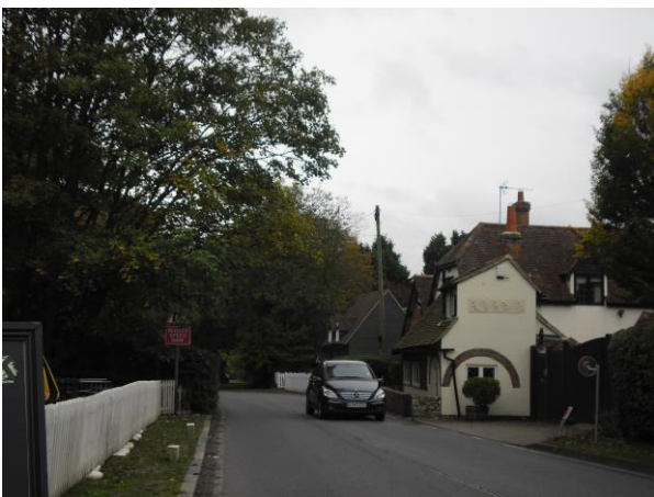
Image 1 – View travelling eastbound along Coopersale Street, bend sign obscured (adjacent to Theydon Oak PH)
